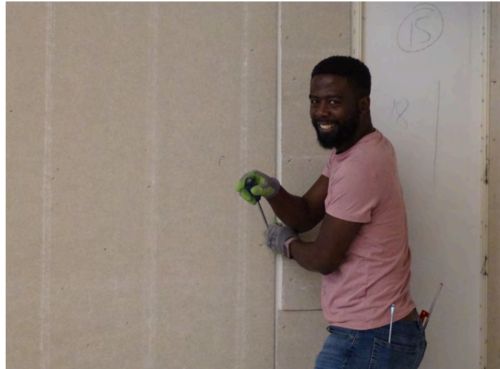
Eric removing old soundproofing
